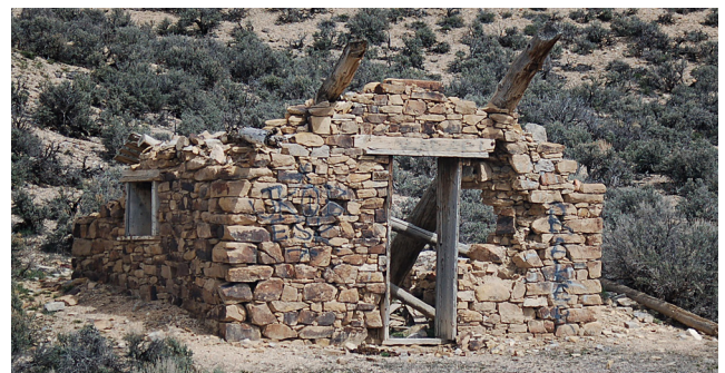
Rosevear Ranch Ruin on Highway 50. Photo by Matt Bowers.
