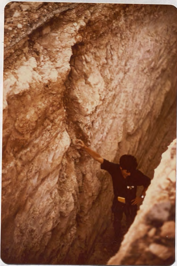
Figure A1-11. One of three normal faults cutting through red and green sandy strata on Brooks Ave, section 15adb, T20S-R61E. Displacement on upper red stratum is approximately two feet.
